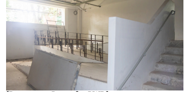
[Basement - Ramp for PWD]
