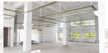
[Fifth Floor - Multipurpose Hall]
